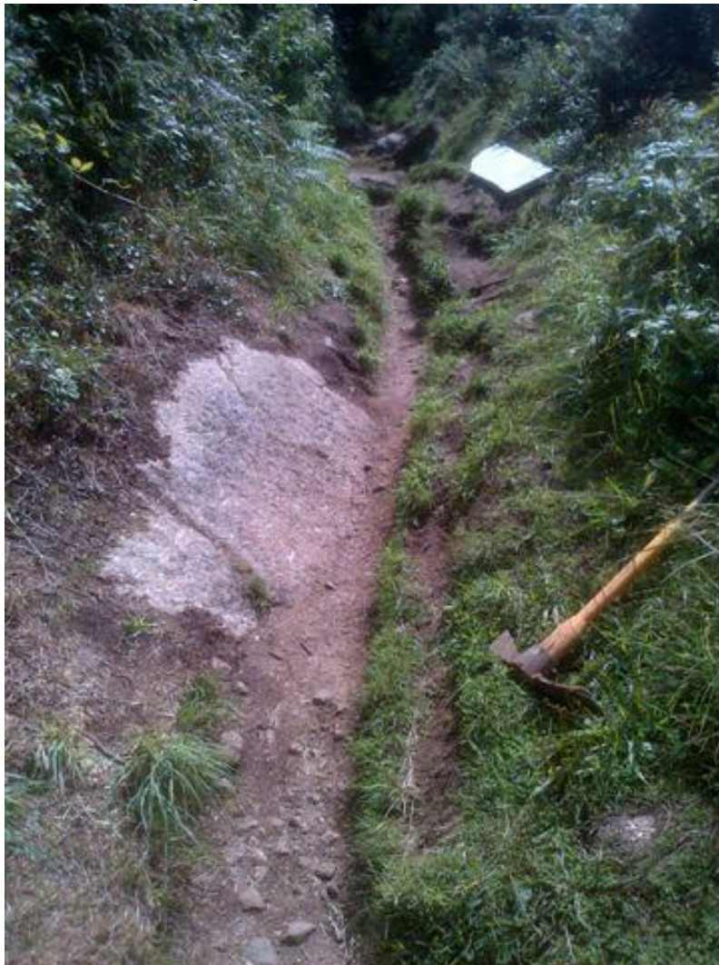
The path before work was started
