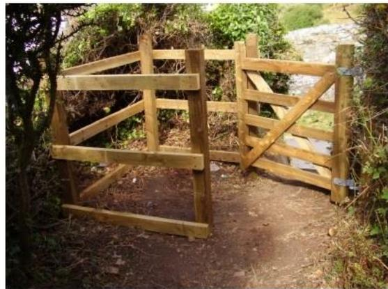
The landowner had been making an attempt to keep this gate usable over the years by tying it together with chains and string. The enclosure area was also overgrown and not very big. We have replaced this with a new kissing gate with room for walkers with big rucksacks and have cleared the vegetation from around here.
