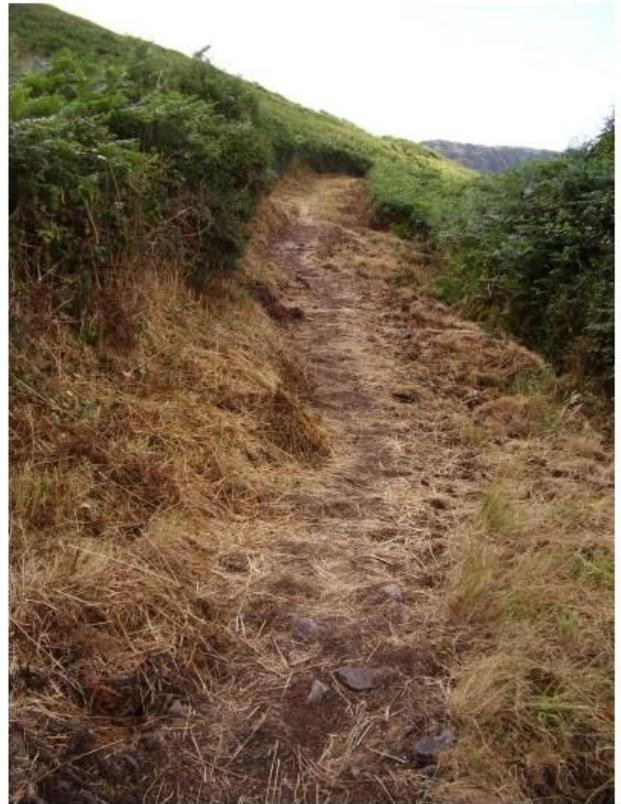
While undertaking a survey of the path, it was noted that there was a particularly rough section of terrain with what appeared to be a large open ditch to the seaward side. A new path was cut approximately 1.5 metres inland to keep walkers away from the ditch. The ground was levelled out and a number of steps were installed at the start of this section to counterbalance the change in levels.
