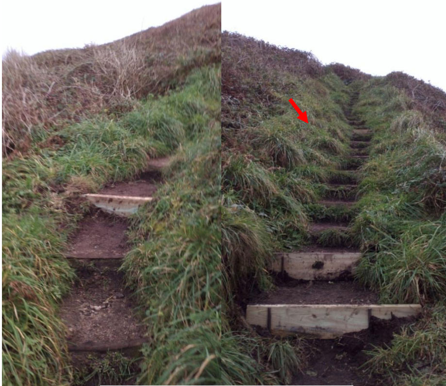
E.7x replacement timber steps
