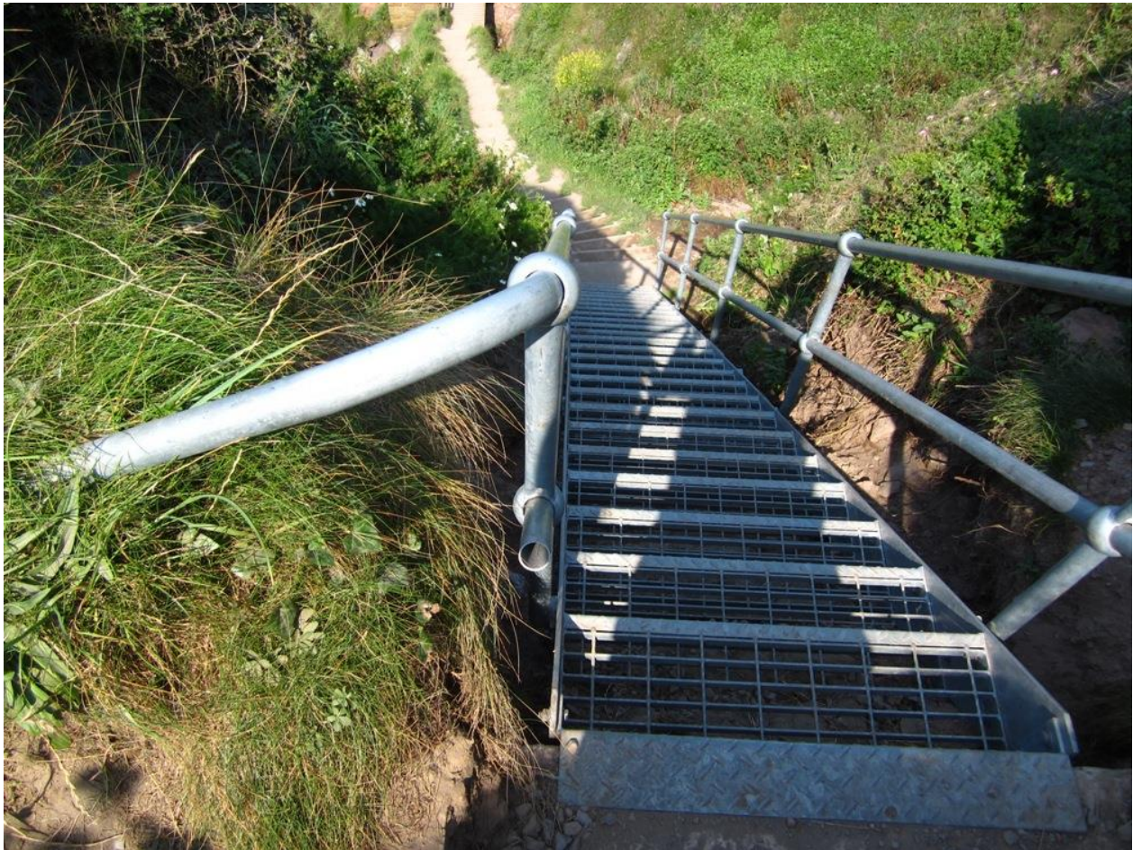
Sharrow steps on completion showing handrails and improved tread construction
