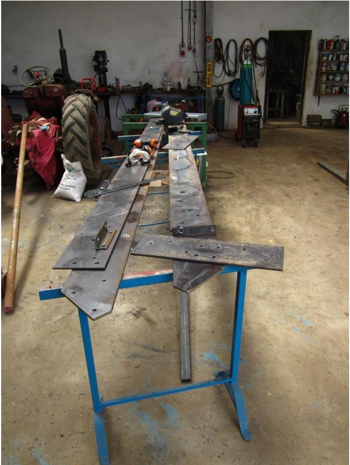
Steps during fabrication
