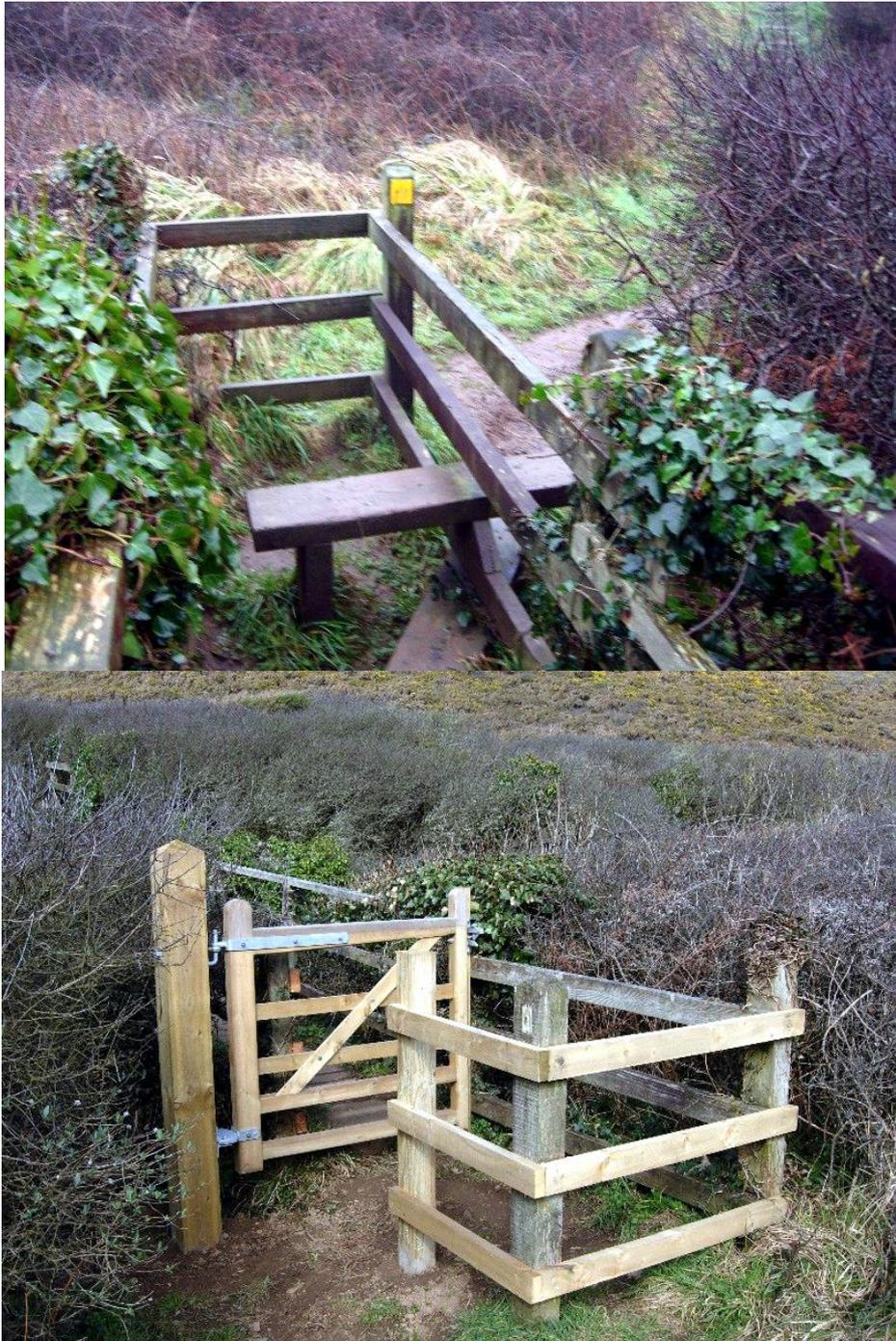
Before and after – the replaced stile and the new kissing gate on the Blegbury/ Blagdon boundary.
